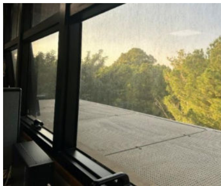
Figure 16: Windows and exterior sunshades
