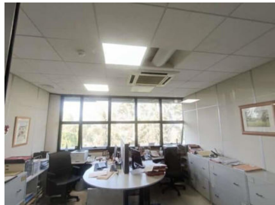
Figure 15: Office frames and lighting fixtures
