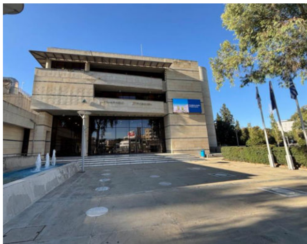
Figure 1: Front View of the Building
