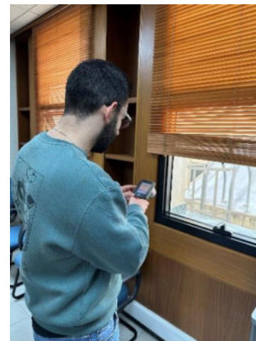
Figure 26: Eastern office window frame (14:05)
