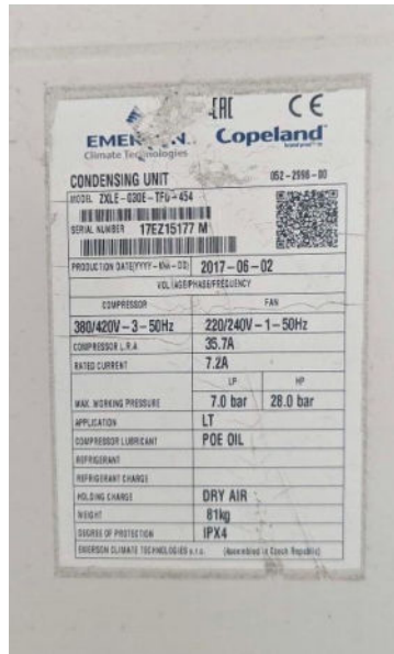
Image 4.3.4d. Technical Specification Cold Room
