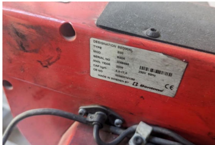
Image 4.4.2b. Technical Specification of Burner
