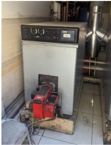
Image 4.4.2a. Diesel Boiler
